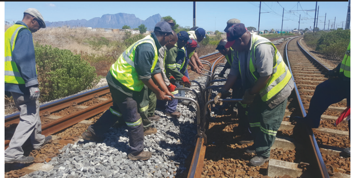
ON THIS PAGE: Employees in Metrorail's perway department have been working diligently to replace worn tracks in Area Central.
