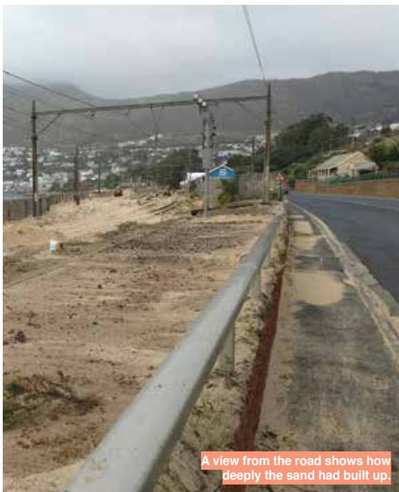
Sand covering tracks between Fish Hoek and Simon's Town stations.
