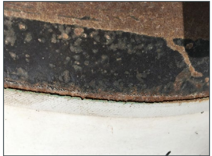
Figure 3b: End disbondment on a pipe with the FBE toe disappeared
