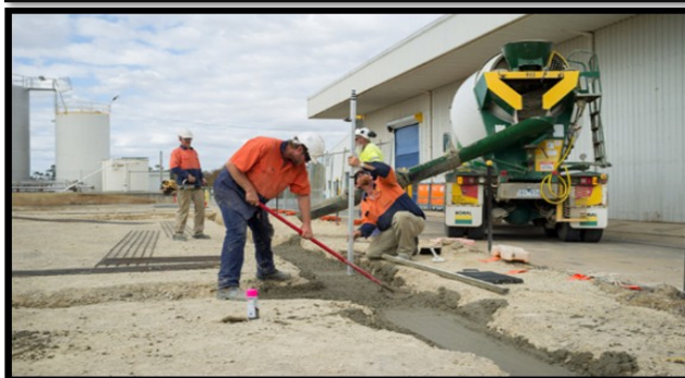
Digging the footings and pouring concrete
