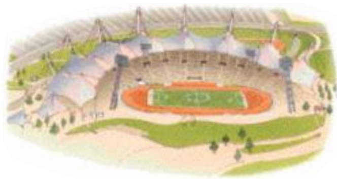
The Olympic stadium in Munich, Germany, built for the 1972 Olympic Games, has a self-cleaning glass roof.
