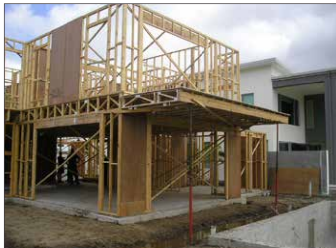
Plywood Bracing - requires onsite installation
