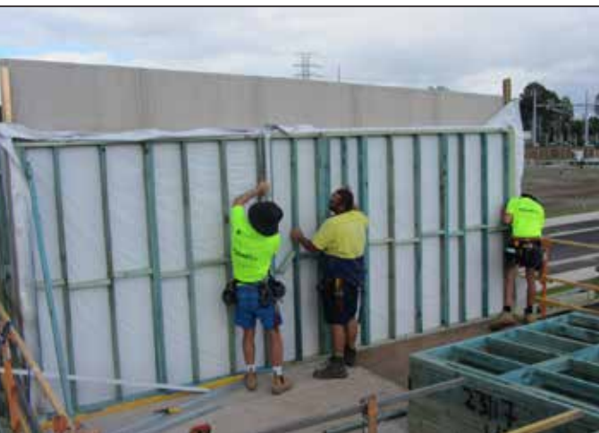
Erecting Boundary Walls
