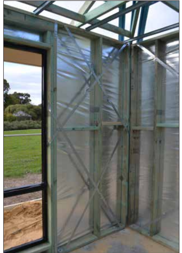
Narrow wall strap bracing unit.
