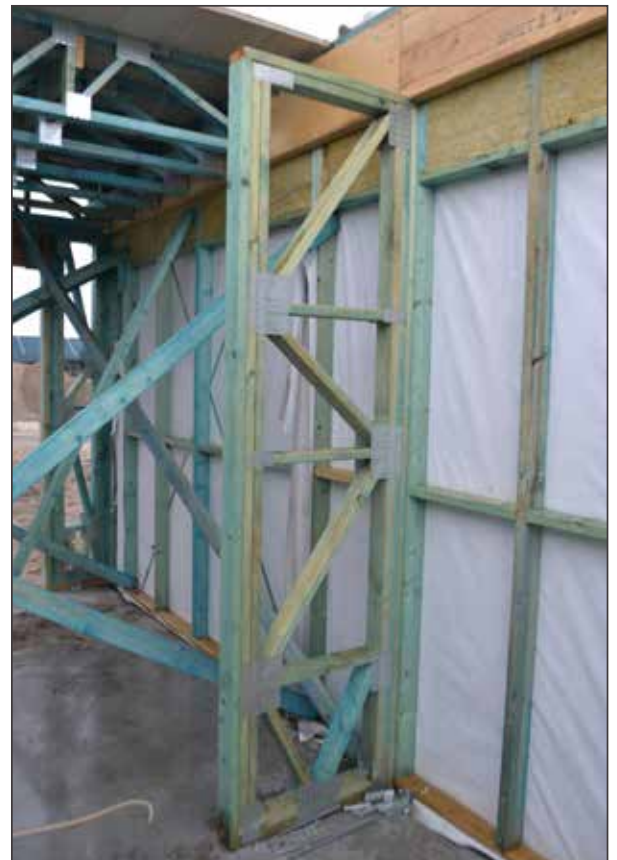
Vertical trussed narrow wall brace.
