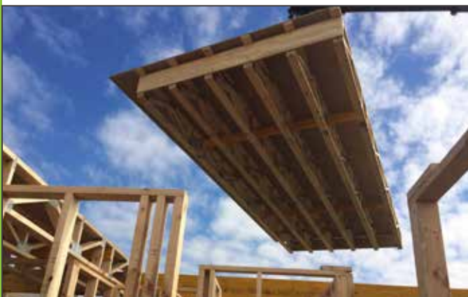
Floor cassette installation
