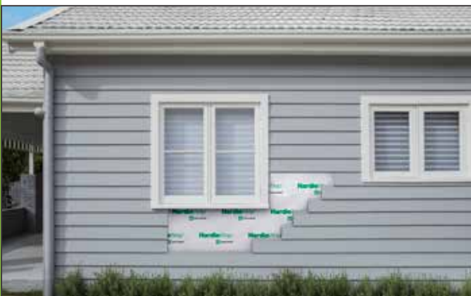
Cut-away of External Cladding to Reveal Membrane Under
