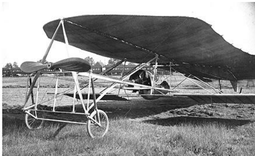
McCORMICK-JAMES "MUSTARD PLASTER" MONOPLANE - CICERO FLYING FIELD - NOVEMBER 1911 DESIGNED BY SIDNEY V. JAMES, FUNDED BY HAROLD F. MCCORMICK - NOTE ROUNDED PARASOL-TYPE REVERSE CAMBERED WING, POWERED BY GIGNE 50 H.P. ROTARY ENGINE DRIVING PARAGON PROPELLER - CARROLL F. GRAY AERONAUTICAL COLLECTION
