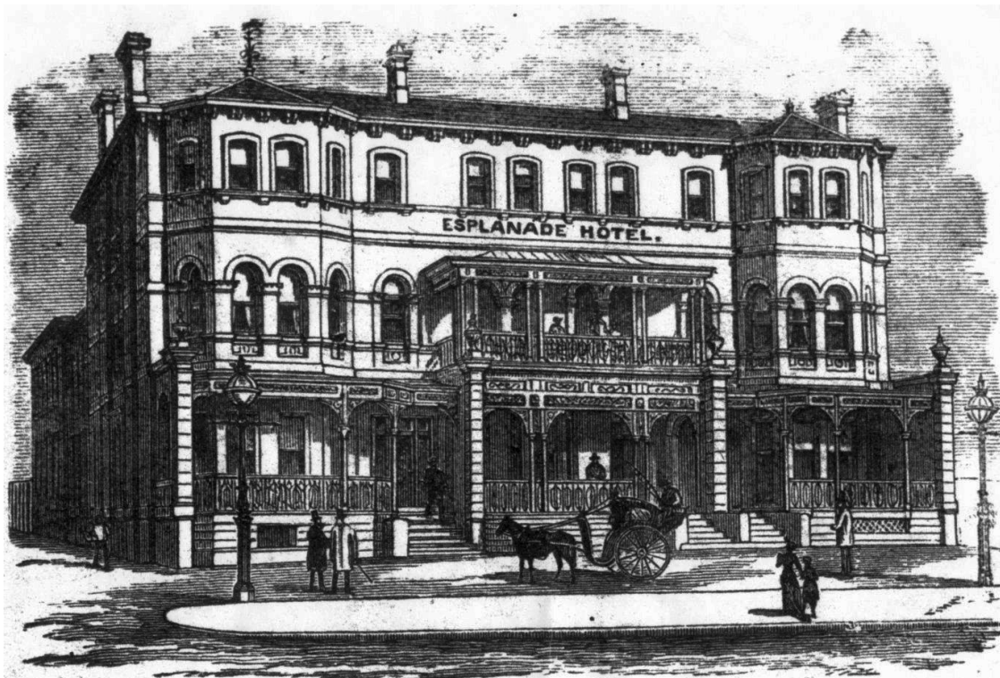
Esplanade Hotel in 1881 showing the three former terraced houses.
