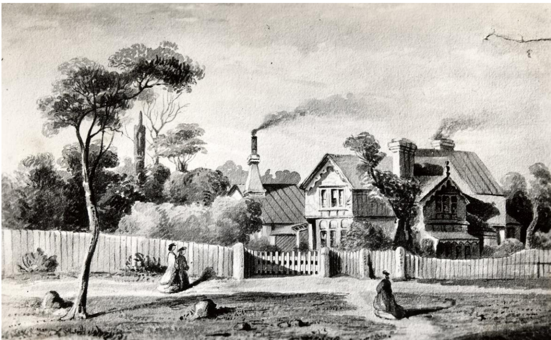
Wattle House, St Kilda, c1865-c66, artist unknown [not Von Guerard], drawing with wash, State Library of Victoria, clearly showing the Morewood & Rogers' iron roof tiles
