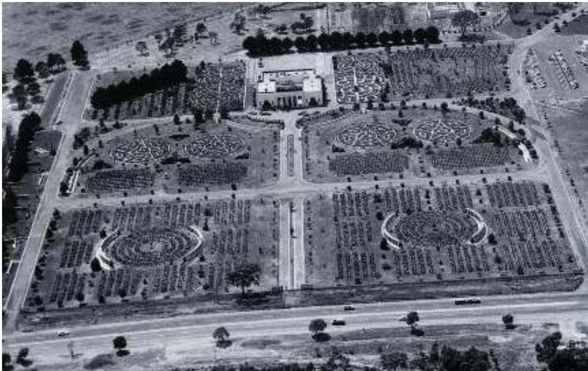
Springvale Crematorium, c1958, Chambers, from Graeme Butler 080618. Above and below.
