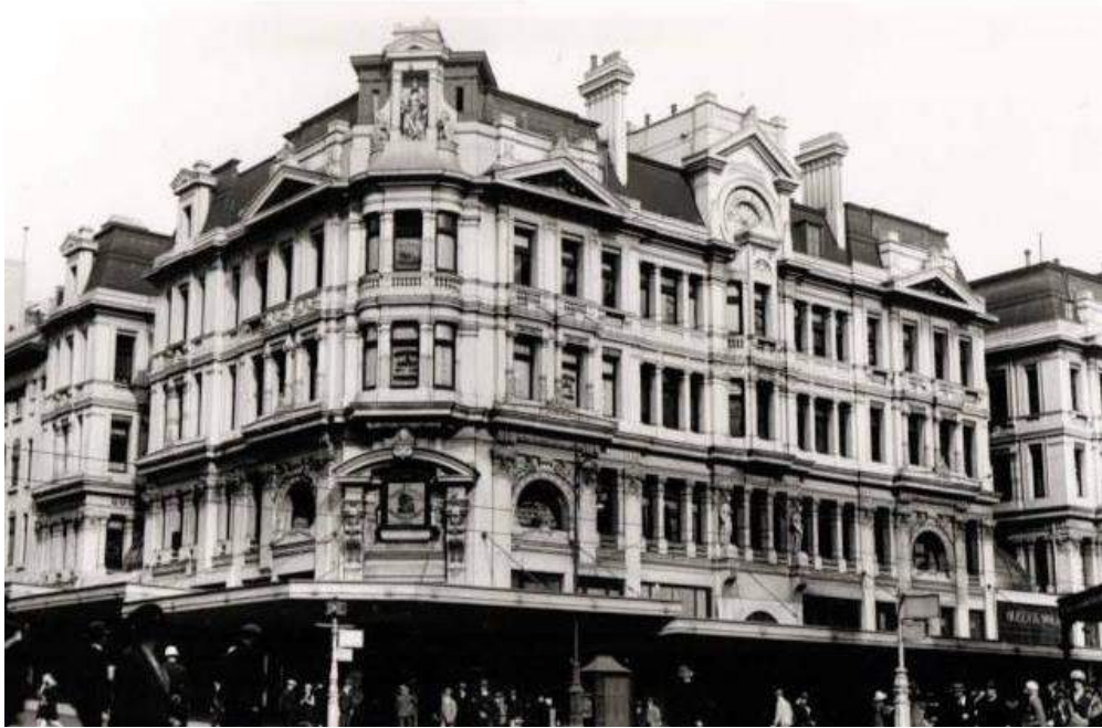
Queen Victoria Building, corner Collins & Swanston Streets, demolished for the City Square.
