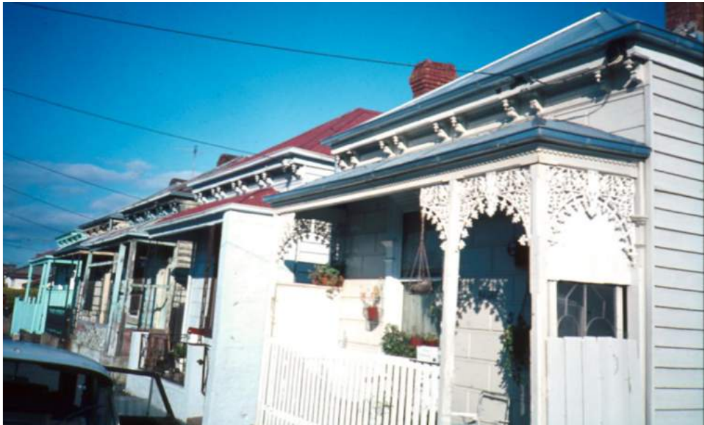
Detached timber workers' houses on The Flat, Park Street, Abbotsford.
