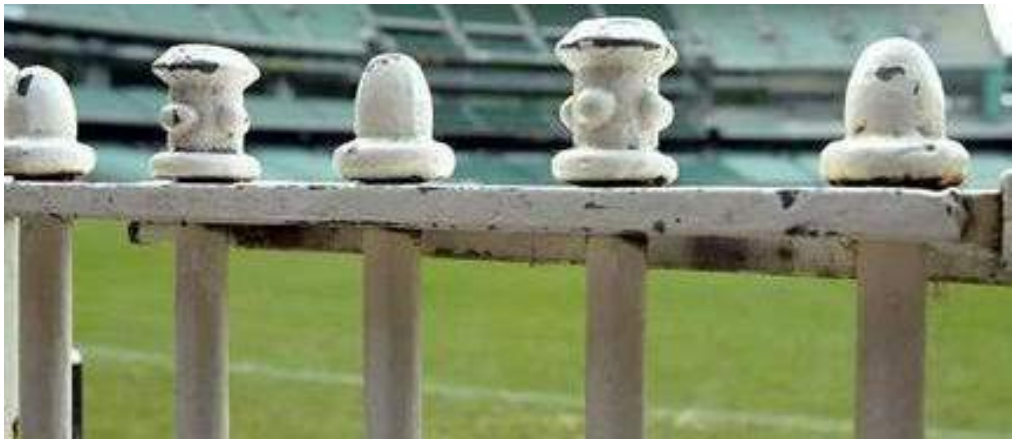
The MCG 1882-83 cast-iron fence, which we would run down towards to see better. Some of it remains in front of the Great Southern Stand around the beginning of the two 50-metre arcs, in front of sections M10 - M13 and M18 - M27. The fleur-de-lys spear-heads were sawn off to modernise it for the Games. A similar fence is at Maddingly Park, Bacchus Marsh.
