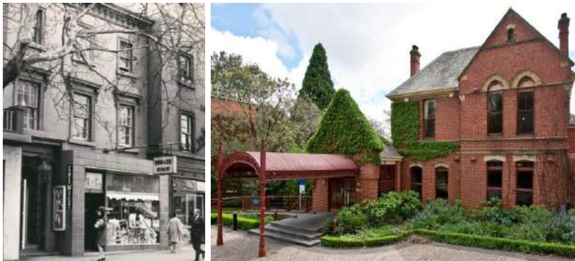
The refurbished Ogg's Pharmacy and University House. The decoration above the canopy has gone and been replaced with a new cast-iron lace valance below.
