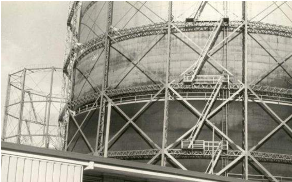
The Gas Works storage cylinders of the Collingwood, Fitzroy & District Gas & Coke Company.
