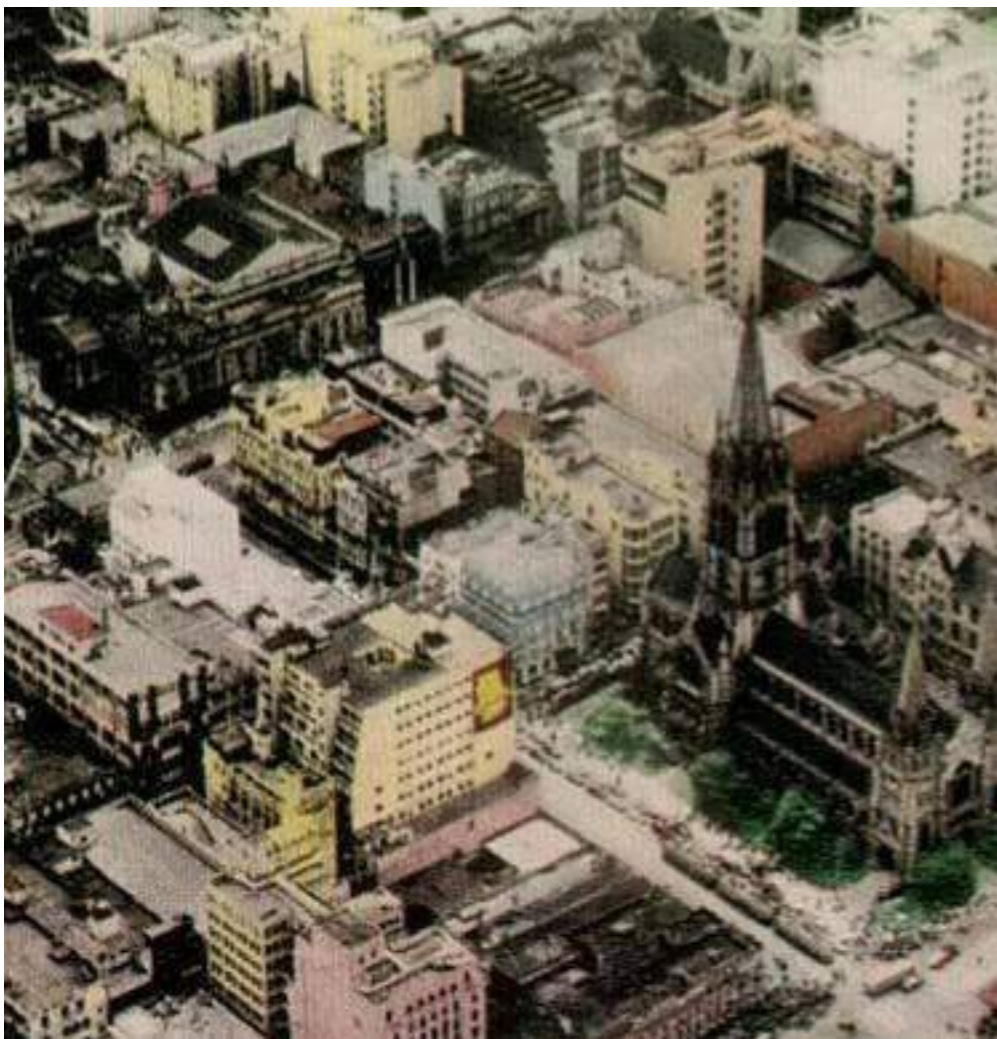
The site demolished for the City Square corner Collins & Swanston Streets.
