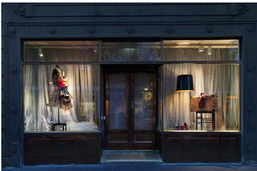
Lilian Wightman's Le Louvre (1932-92), the famous salon of Paris fashion (1940s-), the only surviving of a terrace of four 1855 townhouses, the polished copper shopfront from 1927, the upper façade and interior Georgianised after 1954. The window display was changed daily, closely watched for by Geoff and me. The business is now at 2 Daly Street, South Yarra www.lelouvre.com.au/#!/the-story/cpeg
