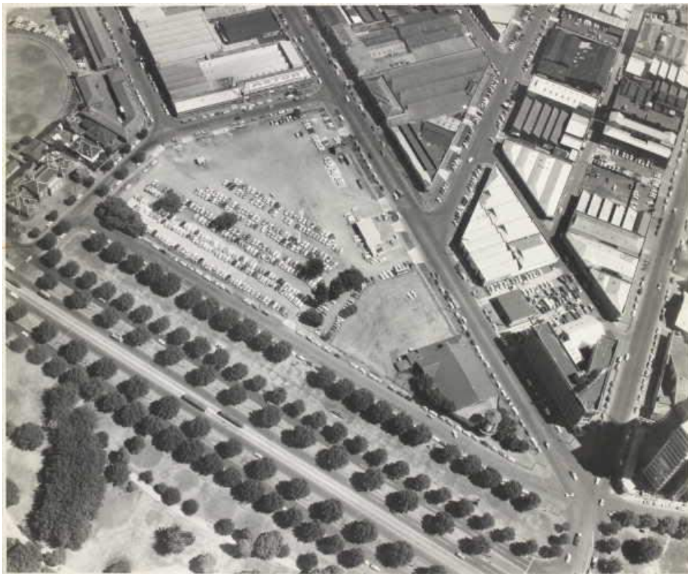
The V-shaped YMCA building is lower right. In the foreground is St Kilda Road and the large triangular site is reserved for the National Gallery of Victoria and the Victorian Arts Centre. The building at its pointy end is the Green Mill Dance Hall.
