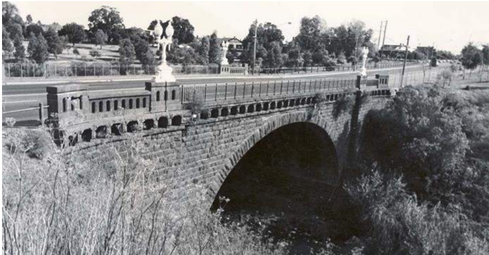
Merri Creek bridge, Heidelberg Road, 1853, bluestone, undated photograph, c1950s?
