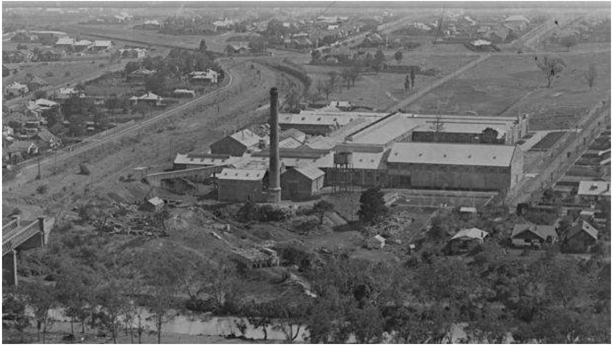
The APM site, 1920s. Heidelberg Road runs from top left to top right. The chimney was the only one of these buildings to survive, perhaps and now that has been recently demolished. The Outer Circle Rail line still exists, but the Chandler Highway has been run beside it, taking a sharp S-bend to cross its bridge.
