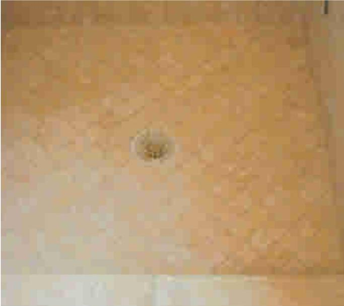
*(Above) Completed shower floor set on a diagonal with plenty of slope to draw the water to the center.*
