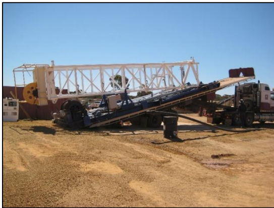
Unloading headframe at the Radio shaft collar
