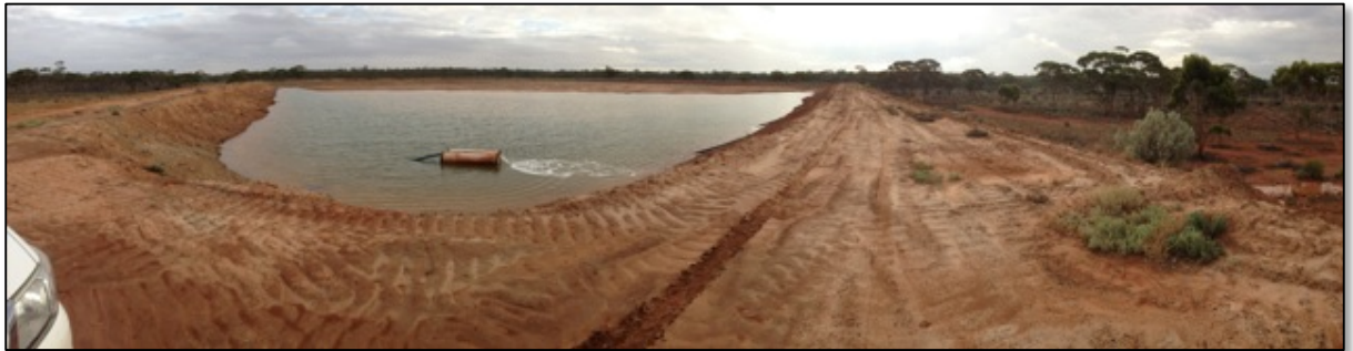
Figure 3 Radio dewatering dam
