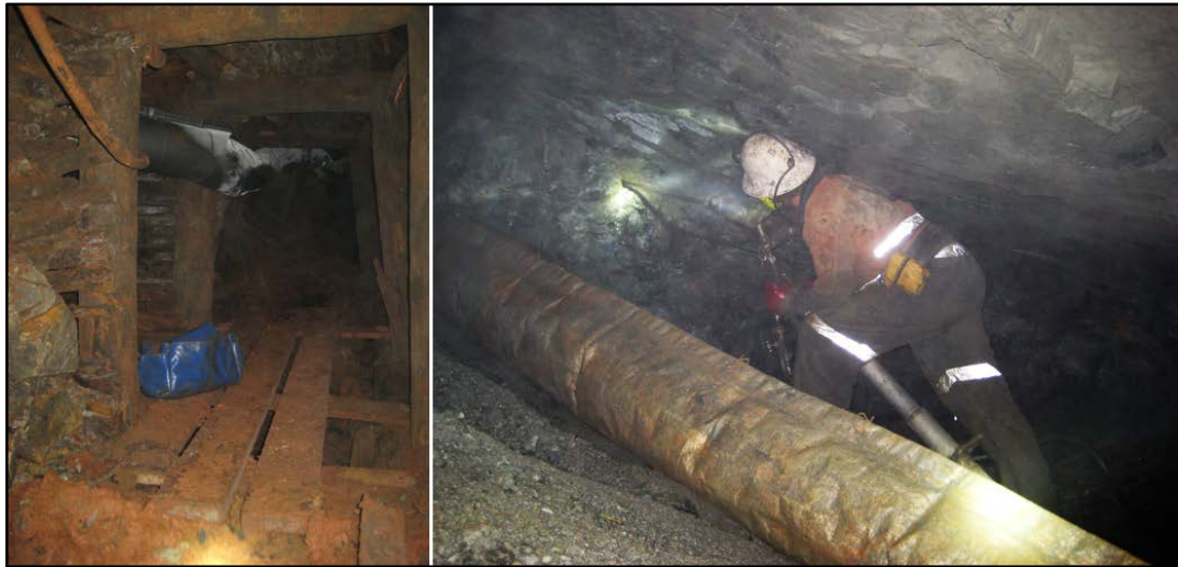
9 Level Underlay shaft crossover
