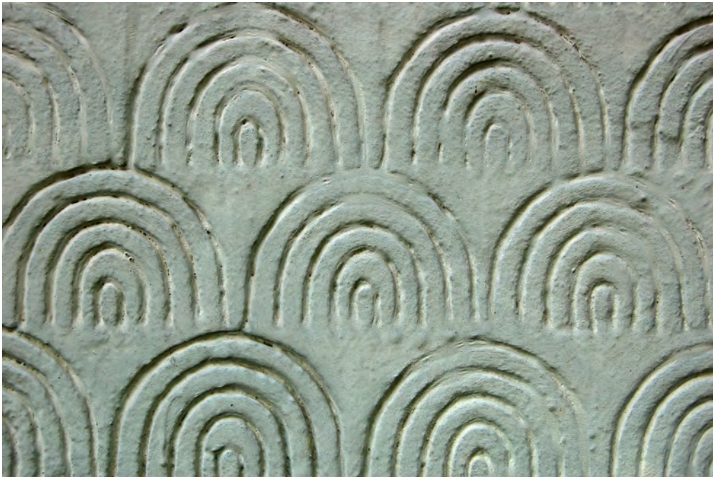
Picture 1.2 Traditional Essex combed pargetting of an unusual almost horseshoe shape on the wall of one of the Rickling Corner Cottages.
