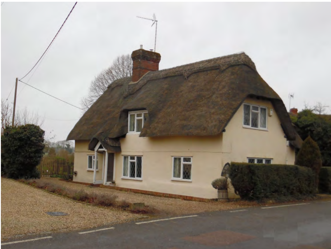
Picture 1.22 Well Cottage: A Grade II listed, thatched cottage on the outskirts of the Green.
