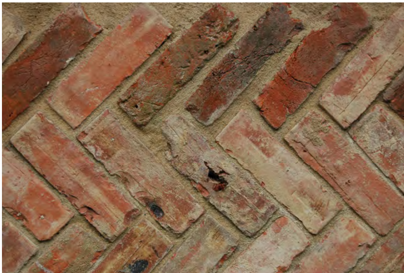
Picture 1.6 Modern brickwork laid in a herringbone pattern is used to good effect in a wall abutting the east side of the Cambridge Road.
