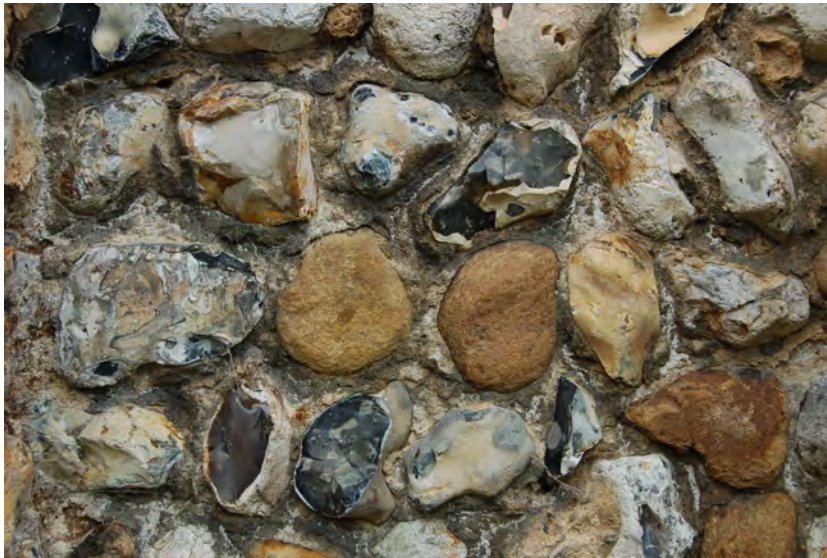
Picture 1.5 Local flint used to good effect in the boundary wall to the church of St Simon and St Jude in Quendon.
