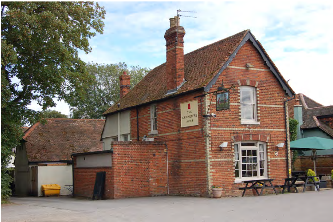
Picture 1.23 The Cricketers Arms public house: A fine 18th century structure with later 19th century alterations enjoying a prominent position overlooking the Green.
