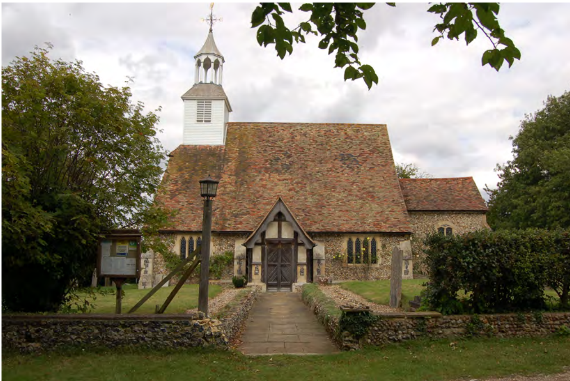
Picture 1.9 Quendon church today with the addition of the timber bell tower which was restored in 2013.
