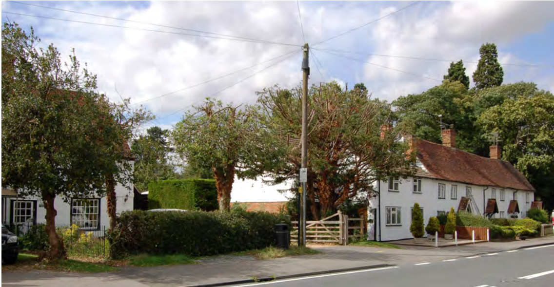
Picture 1.19 Utility poles, particularly in close proximity to quality listed buildings, introduce a discordant element into the street scene. If at all practicable, their replacement with underground services would be a significant improvement.
