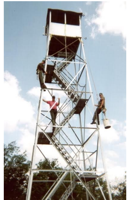
The tower in restoration; Rangers painting the tower, 2003. Photo: NYSDEC
