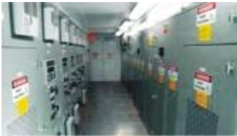
Electric Drive System (VFD/MCC house)
