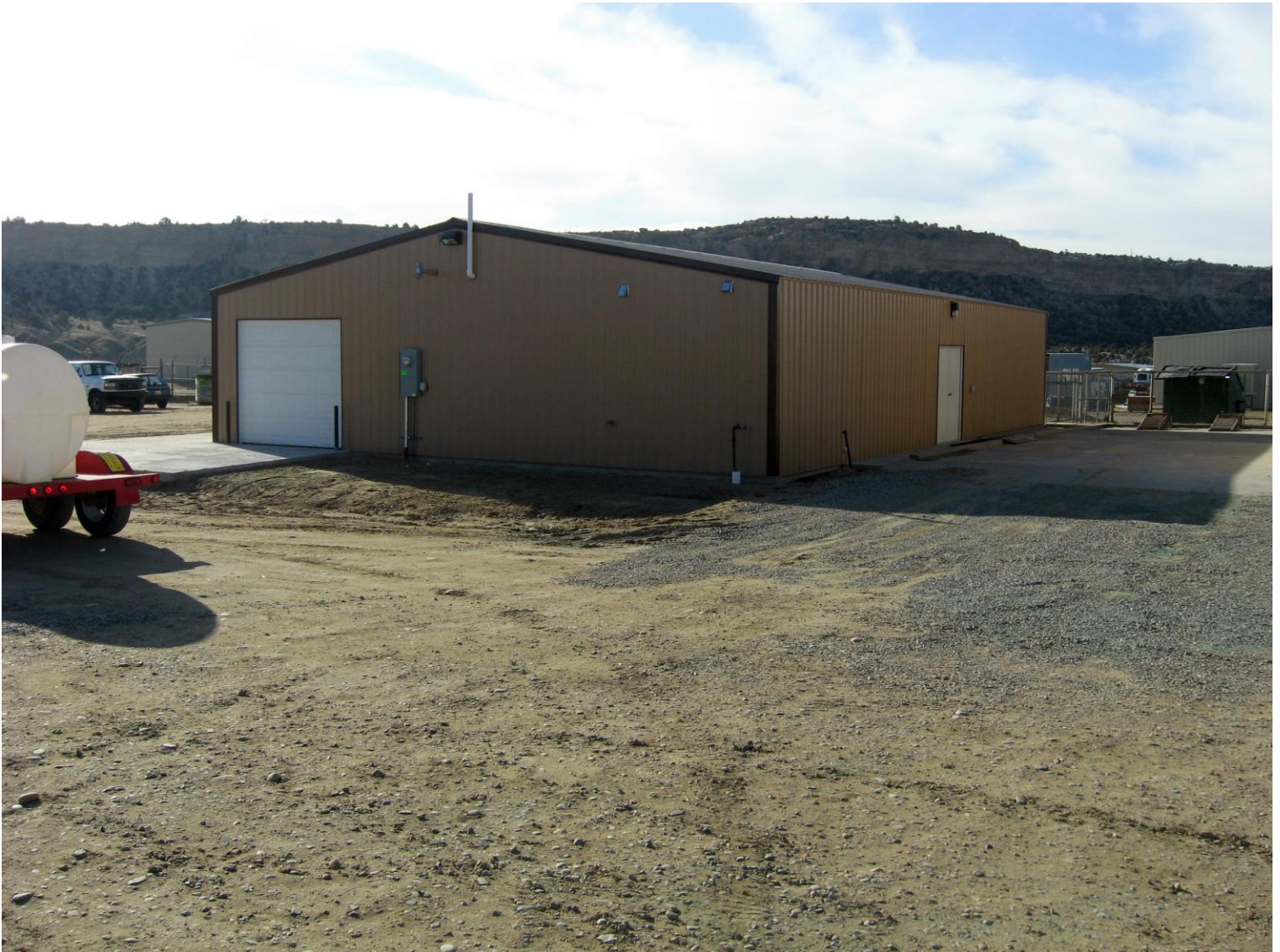
Back of building looking South.
