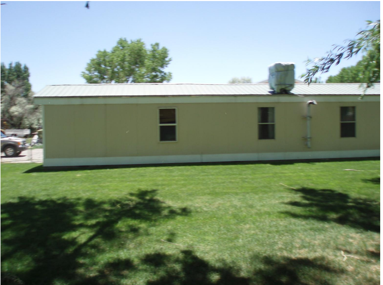
West side of structure 6/06/2012
