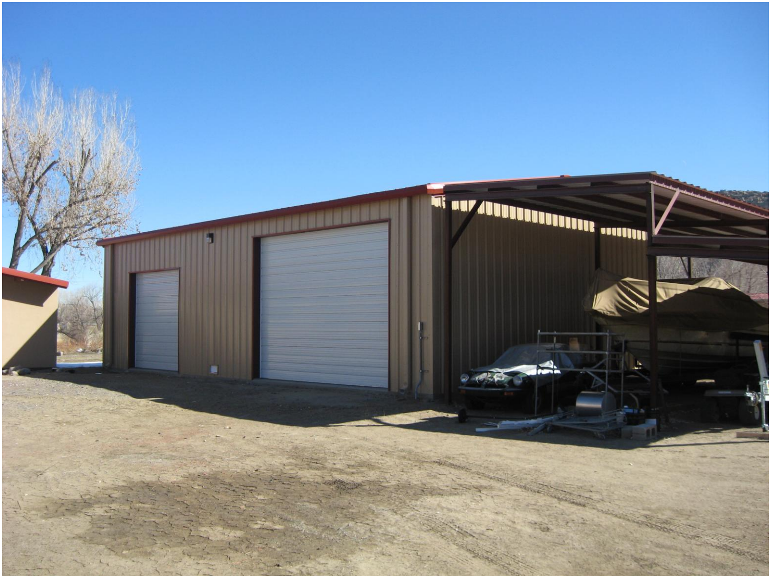
Front of structure looking North 2/15/13
