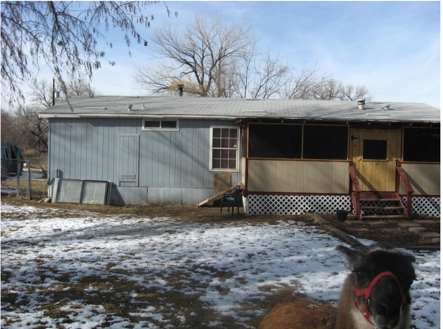
Back of structure looking Norherly
