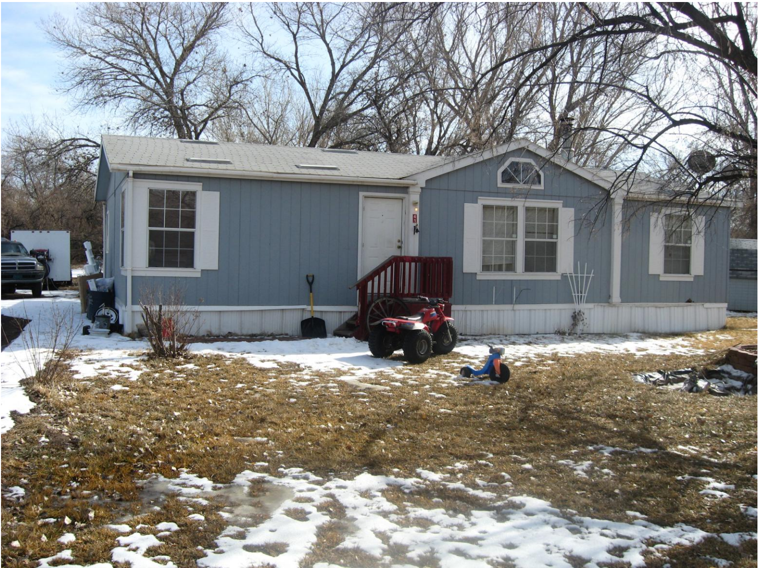
Front of structure, looking Southerly.
