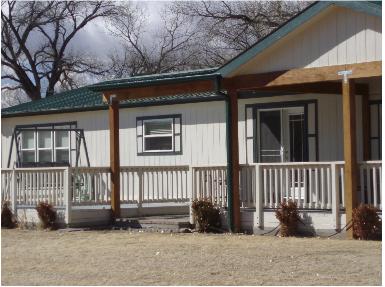
Front of structure looking West 2/26/13
