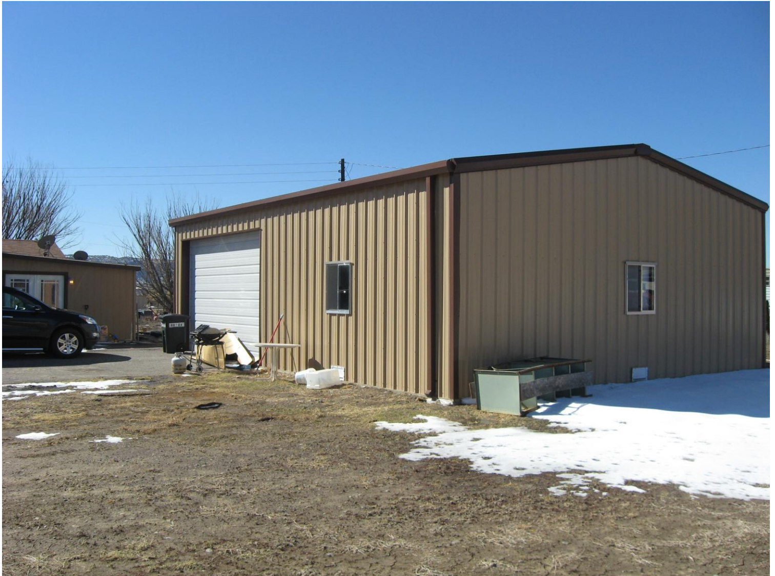
Front of structure looking Northwest 2/15/13
