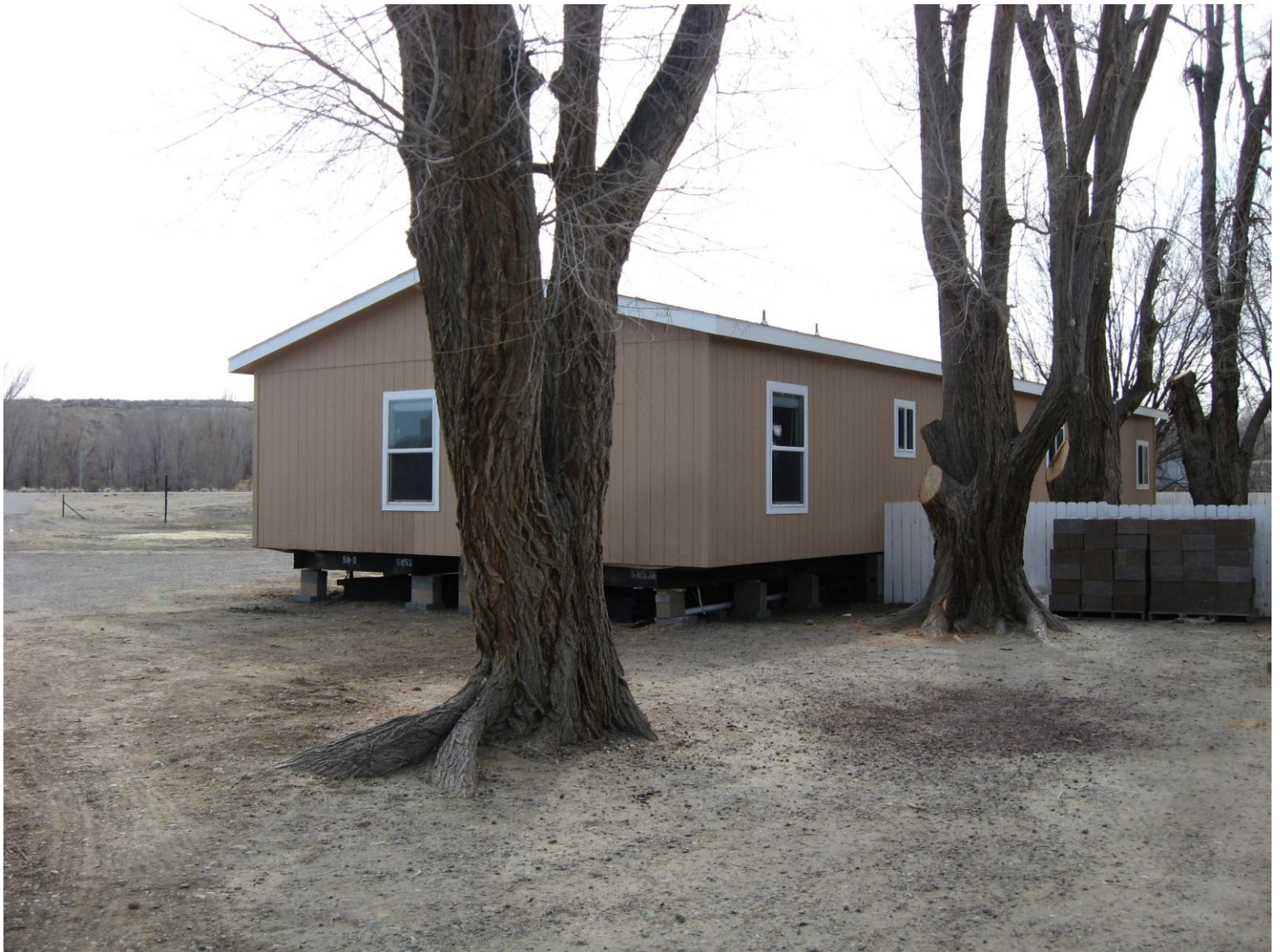
Back and side of structure, looking SW. 3/5/13
