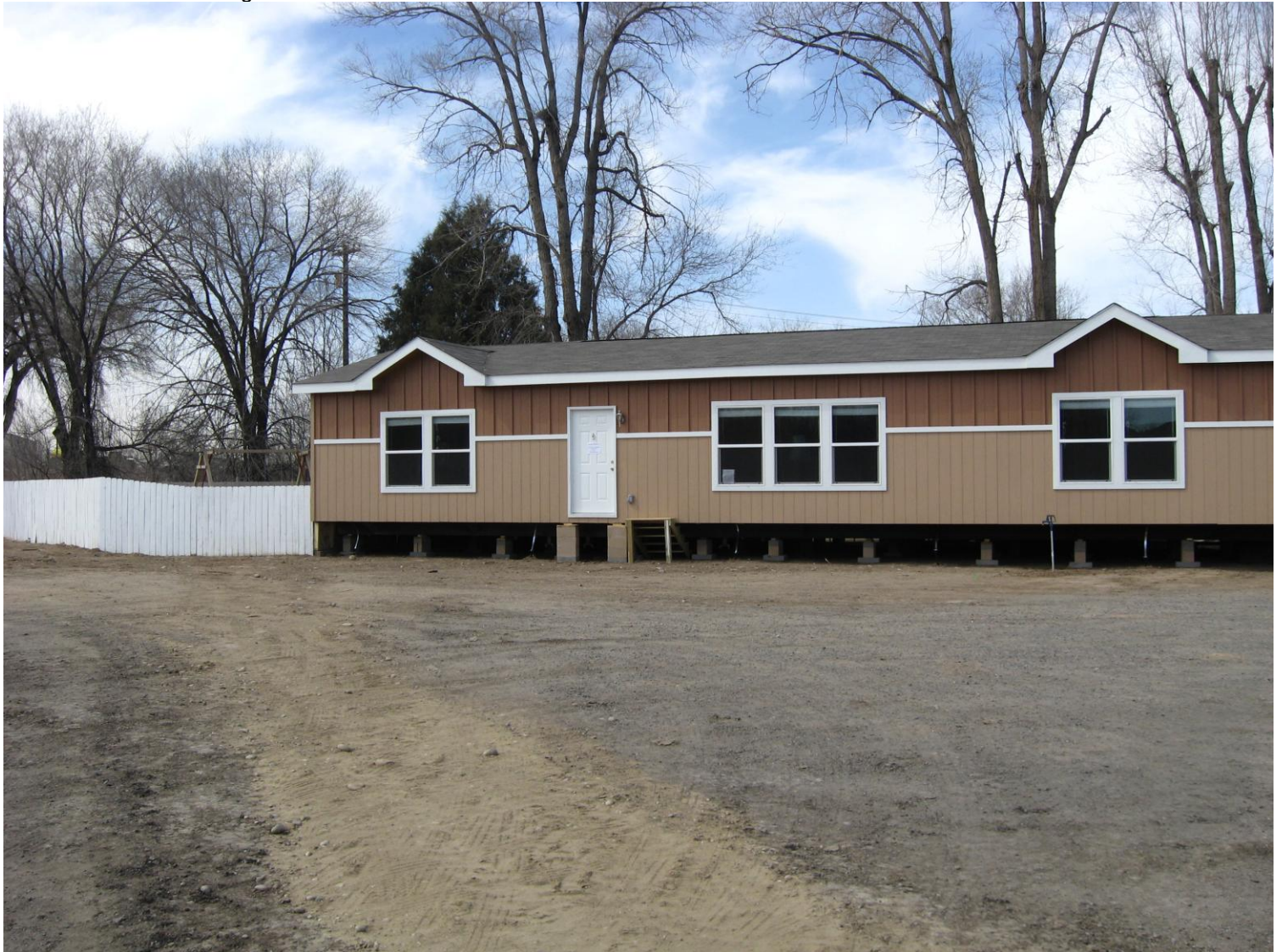
Front of structure looking North. 3/5/13
