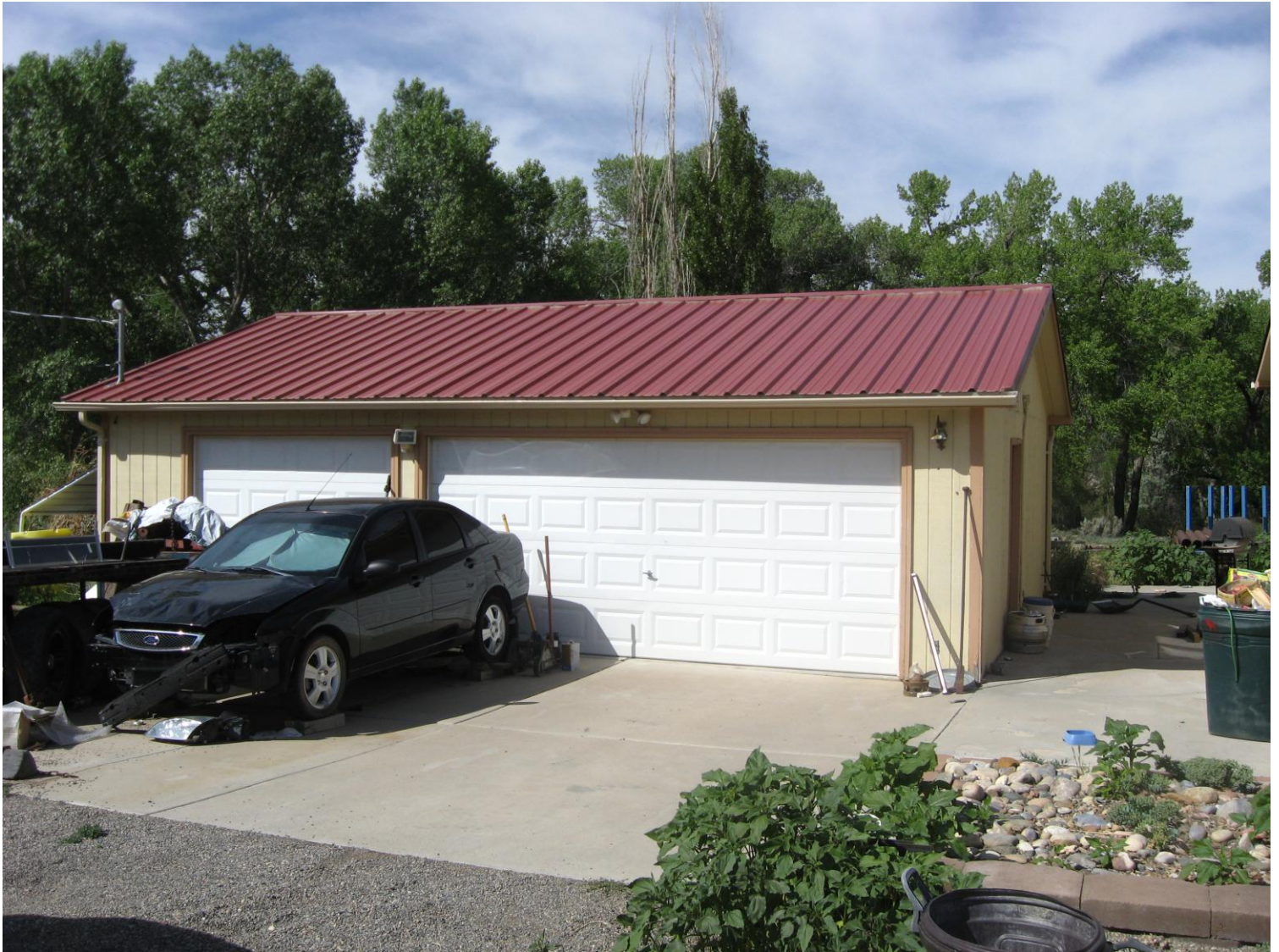
Front of structure looking Southwest 6/2/13
