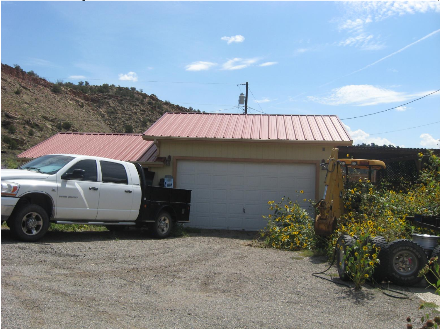
Front of structure looking South 9/9/13
