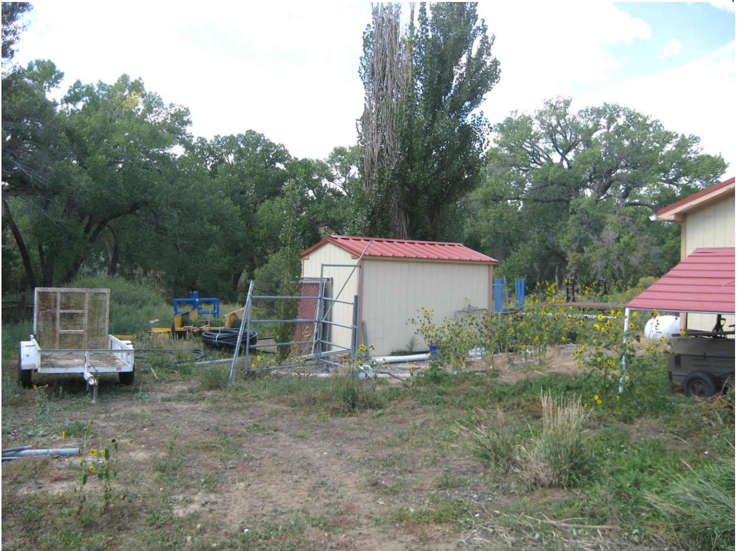
Front of structure looking west 9/9/13
