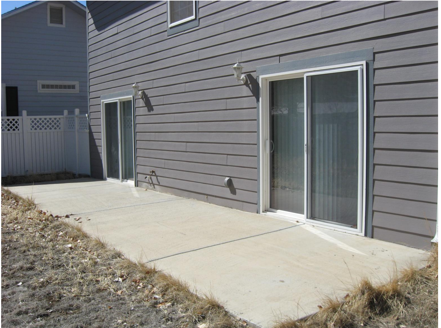
Back of structure looking SW. 3/12/13
