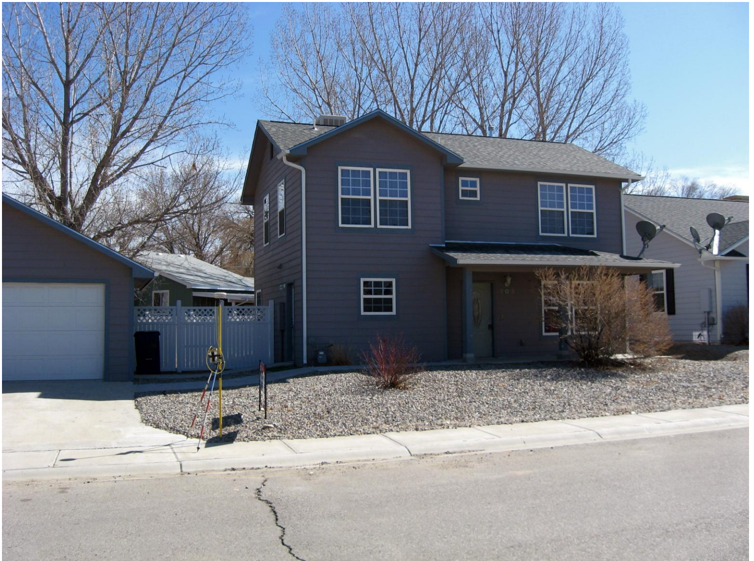
Front of structure looking East. 3/12/13
