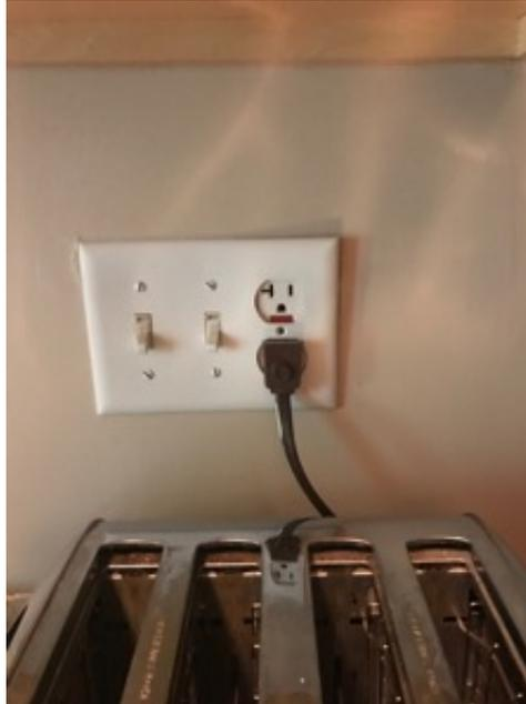
**Three-prong** - Ground plug is broken off in receptacle therefore not allowing a grounded plug to be plugged in. I suggest a certified electrician evaluate further.
