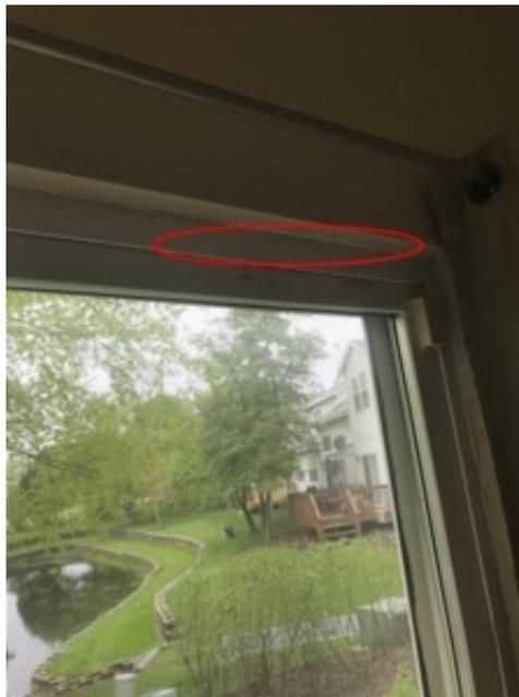
**Window stuck** - Window does not open and close properly and should be repaired.
