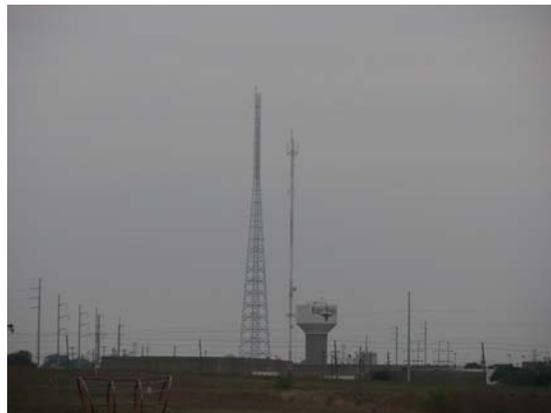
*The new Rolling Hills tower, left, is 80 feet taller than the existing tower.*
