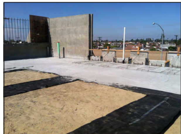
Specially designed ELASTIZELL EF footing pad (six feet thick) for bridge abutment and wing wall. ELASTIZELL EF was also placed about 14 feet thick behind the abutment and wing walls.
