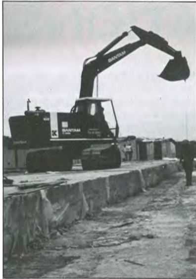
Heavy equipment operates directly on 25 pcf ELASTIZELL EF.
