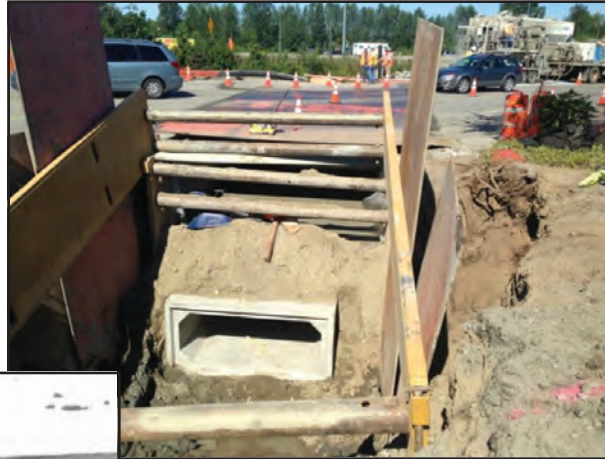
Totem Lake, WA Unacceptable loads on structure
