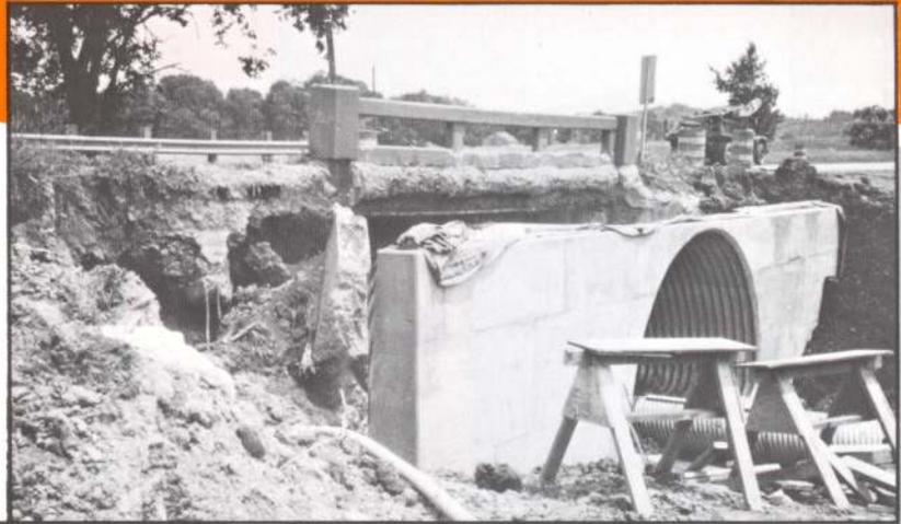
New corrugated steel culvert end walls are placed through the deteriorated bridge.
