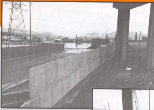
ELASTIZELL EF is placed within two rows of precast containment panels — 6' wide, 6.5' high, 4" thick.
