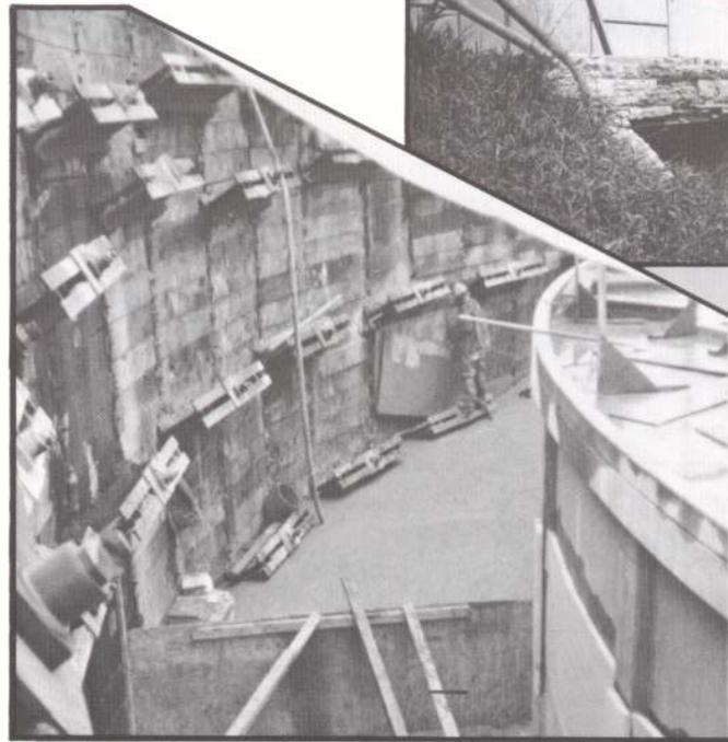
ELASTIZELL EF fills space between tied back wall and partially buried water tank eliminating uneven pressures on tank walls.
