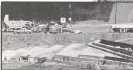
**ELASTIZELL EF** is engineered for load balancing to fit the sloping culvert, the depth of fill over the culvert, and the final ramp elevations.
