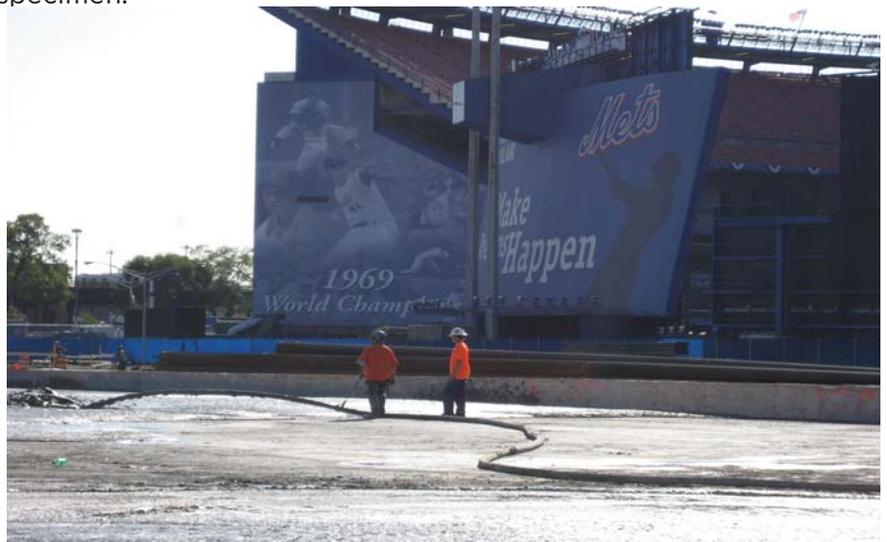
AQUAERiX™ P-CLWC was installed as a sub-base under the playing field at New York's Citi Field to facilitate drainage, replacing the 4 feet of lightweight aggregate listed in the original spec saving the owner time and cost.
