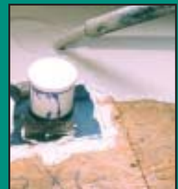
Voids and penetrations in the floor must be carefully sealed before pouring LEVELROCK underlayment.
