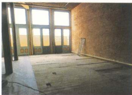
DETERIORATED FLOOR
