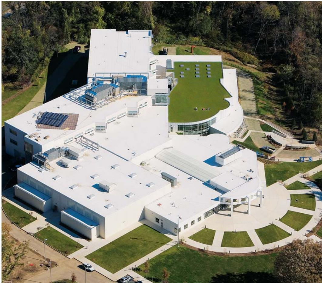
Applied over ZIC Lightweight Insulating Concrete, more than 600 squares of Paradiene 20 TG F/Paradiene 30 CR FR TG provide an energy efficient, bright white cool roof solution for this Philadelphia school. Liquid-applied Parapro 123 Flashing was used on the project. The school's green roof area was completed with Teranap.
