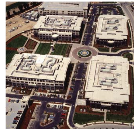
▲ This impressive complex in northern California is protected by a Paradiene 20/30 System installed over Siplast Lightweight Insulating Concrete.
