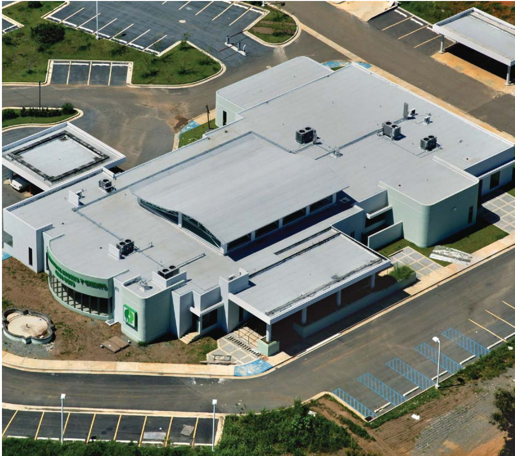
▲ The Insulcel-RT Lightweight Insulating Concrete System and a Paradiene 20 TS/ 30 TG Roof Membrane System were chosen for this bank in Puerto Rico.
