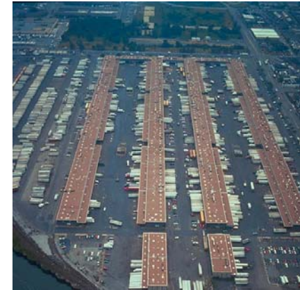
▲ Siplast Lightweight Insulating Concrete and over 7,000 squares of torch grade Paradiene work as a complete system to protect this fruit and vegetable market in the Bronx.
