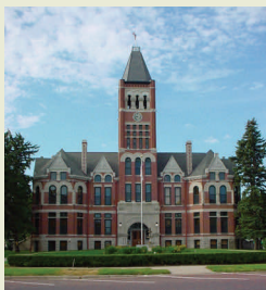
Fillmore County Courthouse
