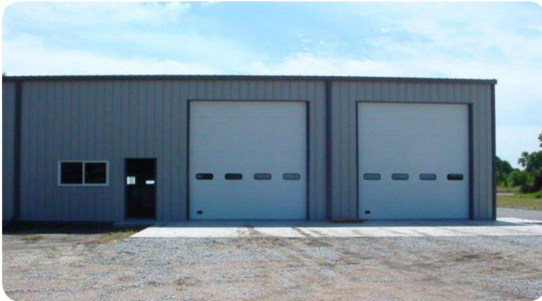
Bill's Repair Shop
