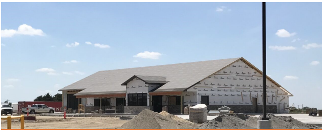
Milligan 41 Express (under construction)
