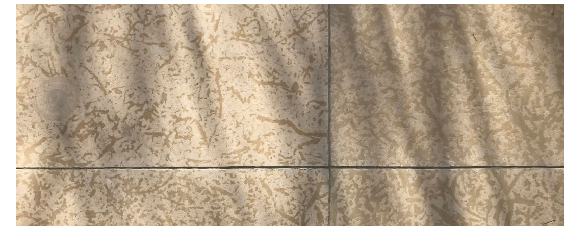
Site photo of the existing Public Safety Building tyndall stone cladding to be recycled into roof pavers
