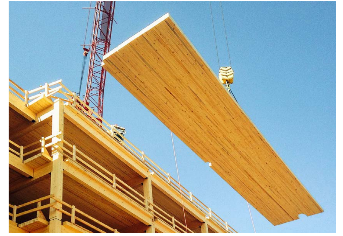
Mass timber construction by StructureCraft (Canada)
