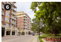
THE EXCELSIOR CONDOMINIUMS 290 Waterfront Dr 48 units
