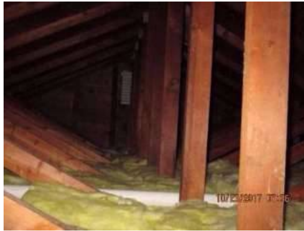
Photo X-24 Attic has batt insulation and is approximately R48
