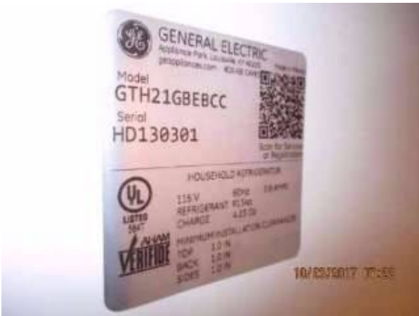
Photo 19-3 Refrigerator data plate.
