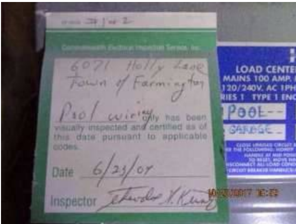
Photo X-13 Stickers showing inspected work in the panel boxes.
