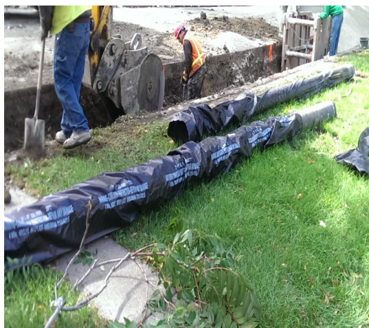
4 MIL Black X-Lam Polywrap Pipe Sleeves Conforms to: ANSI/AWWA C105/A21.5
