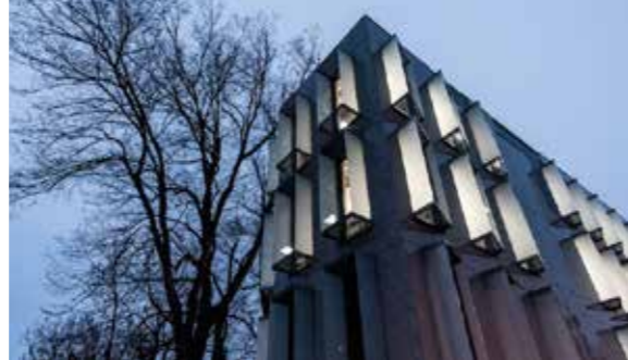
PLATOU CLARKSON OFFICES BUILDING - OSLO (NORWAY)
