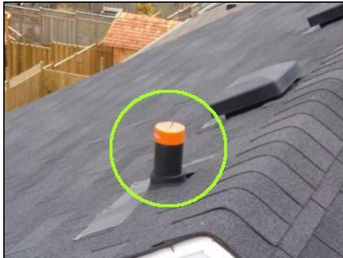
15. Plumbing stack is capped
