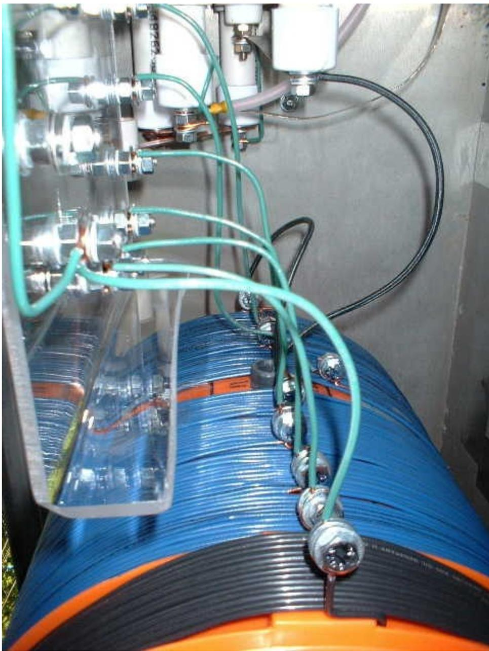
Looking from the bottom of the tuning cabinet behind the coil tap switch, showing the bolted MF loading coil tap connections and the wires running from the MF loading coil to the tap switch. Note the black Variometer coil wires exiting the black shaft pipe near the middle of the blue winding on the loading coil.
