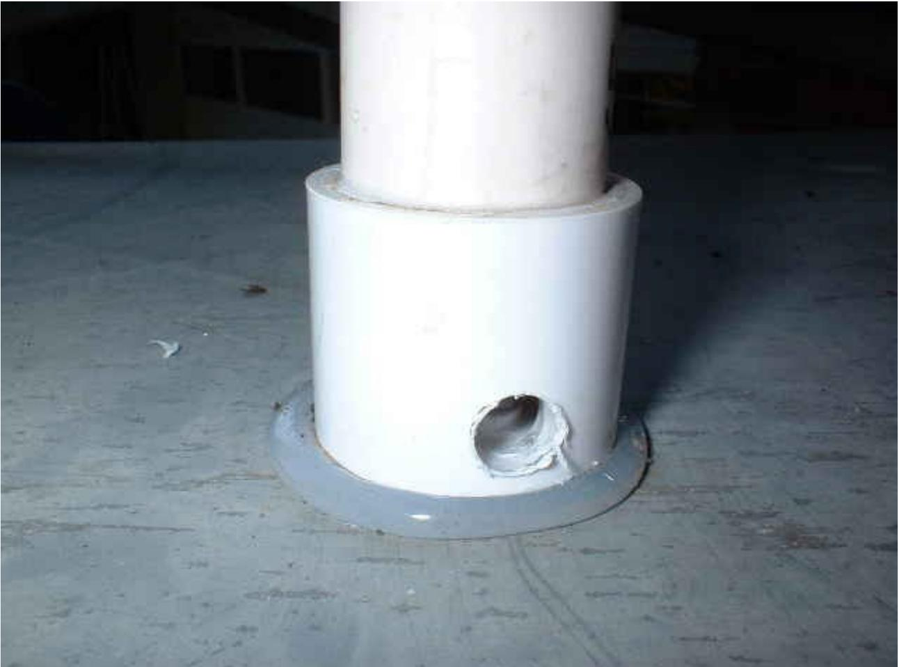
Did you notice that the top ends of the PVC pipe coil support legs were open? That means that they will catch rainwater and may cause leaks into the tuning cabinet. If you use this mounting method, be sure to drill 3/8 inch drain holes in the
