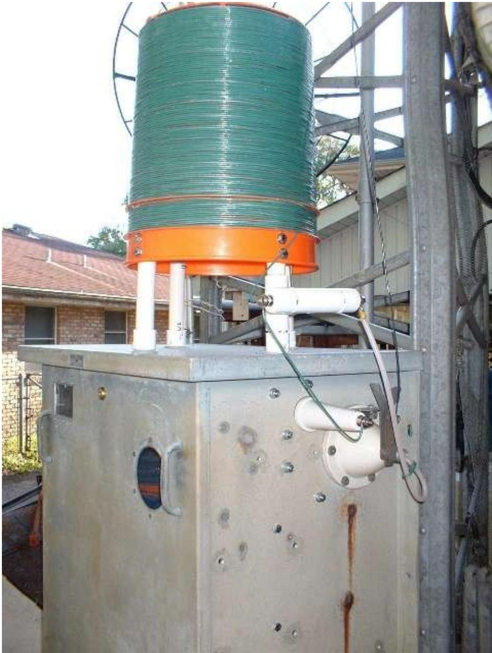
This view shows the LF loading coil mounted on top of the antenna tuner. The loading coil is supported about 6 inches away from the tuning cabinet and the tower. The presence of the cabinet and the tower do not materially affect the operation of the loading coil.
