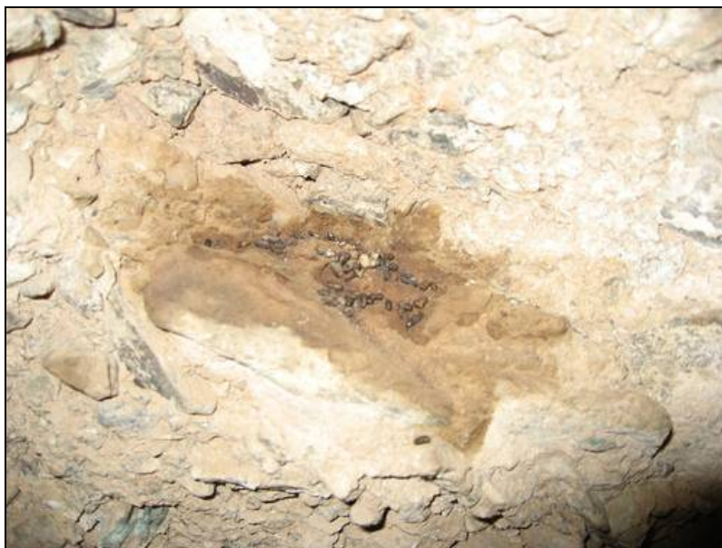
Photograph 8. Possible bat urine staining and guano high on the wall within Adit 5. Photograph date: 22 February 2008.
