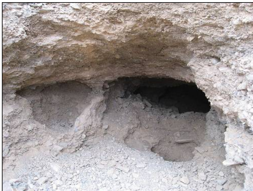
Photograph 3. View at the entrance of Adit 1, looking west. Note the short height of the adit and shallow depth. Photograph date: 22 February 2008.
