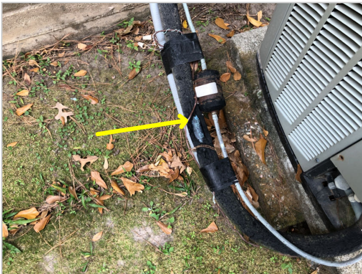
Damaged insulation on AC line. Left side
