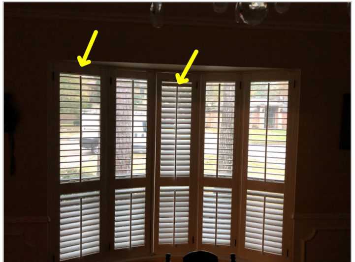
Damaged louver catches
