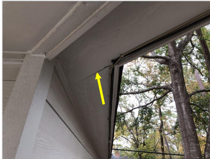
Caulk separation near garage
