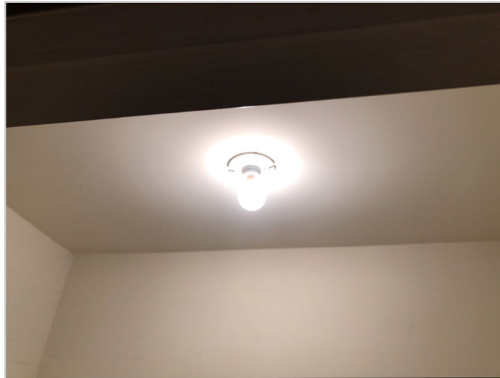
Exposed bulb in closet
