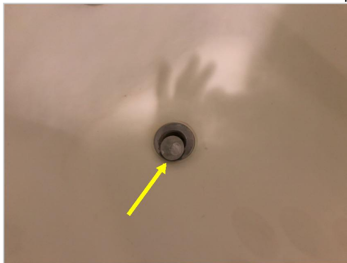
Damaged drain stop
